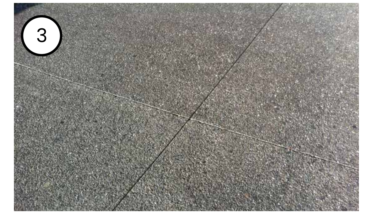
3 Concrete Paving with Exposed Aggregate Finish
