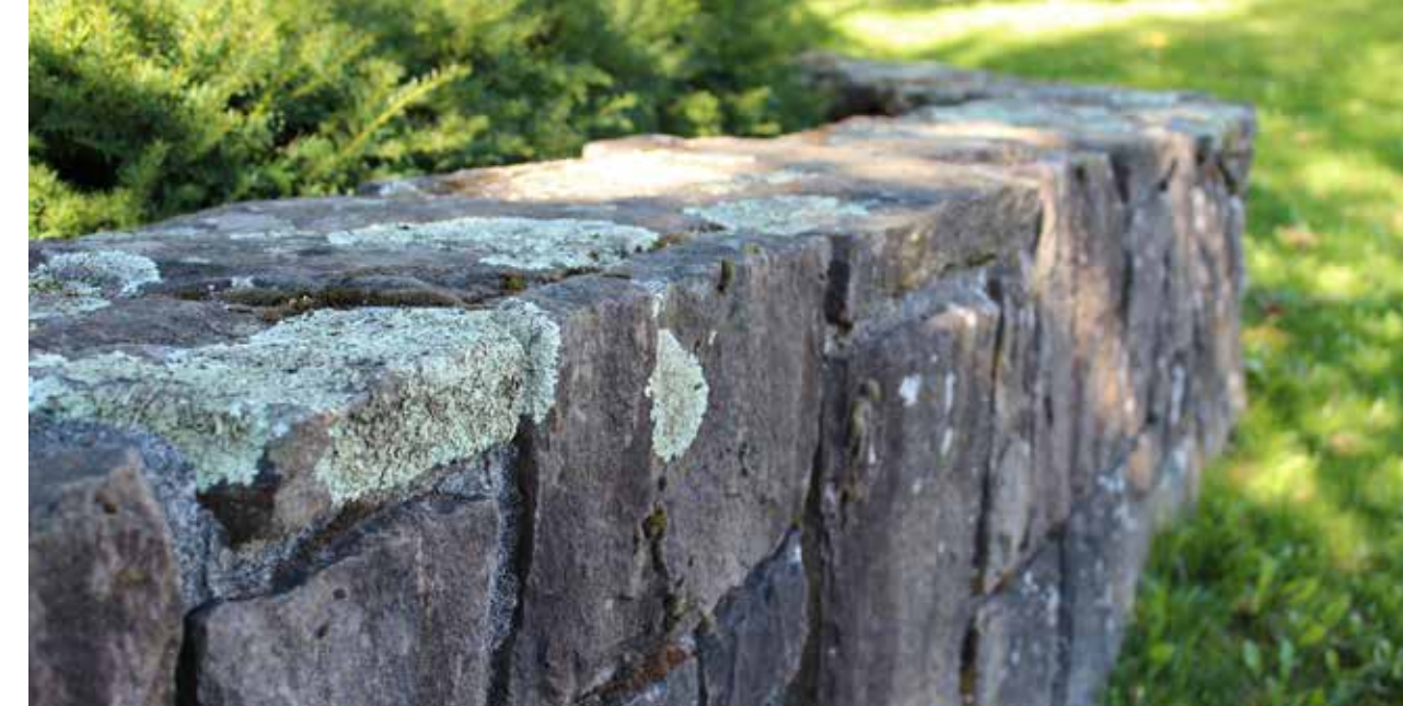
Basalt Ledge Stone Retaining Walls
